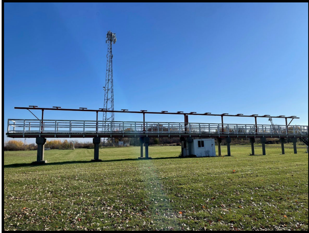
Figure 29: Monitoring and observation installation, eastern portion. (MH1136-D042)
