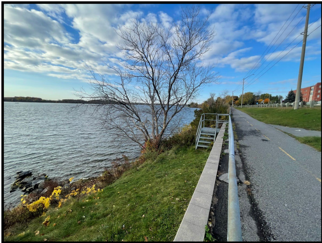
Figure 38: Built-up shoreline between the river and the bike path. (MH1136-D005)
