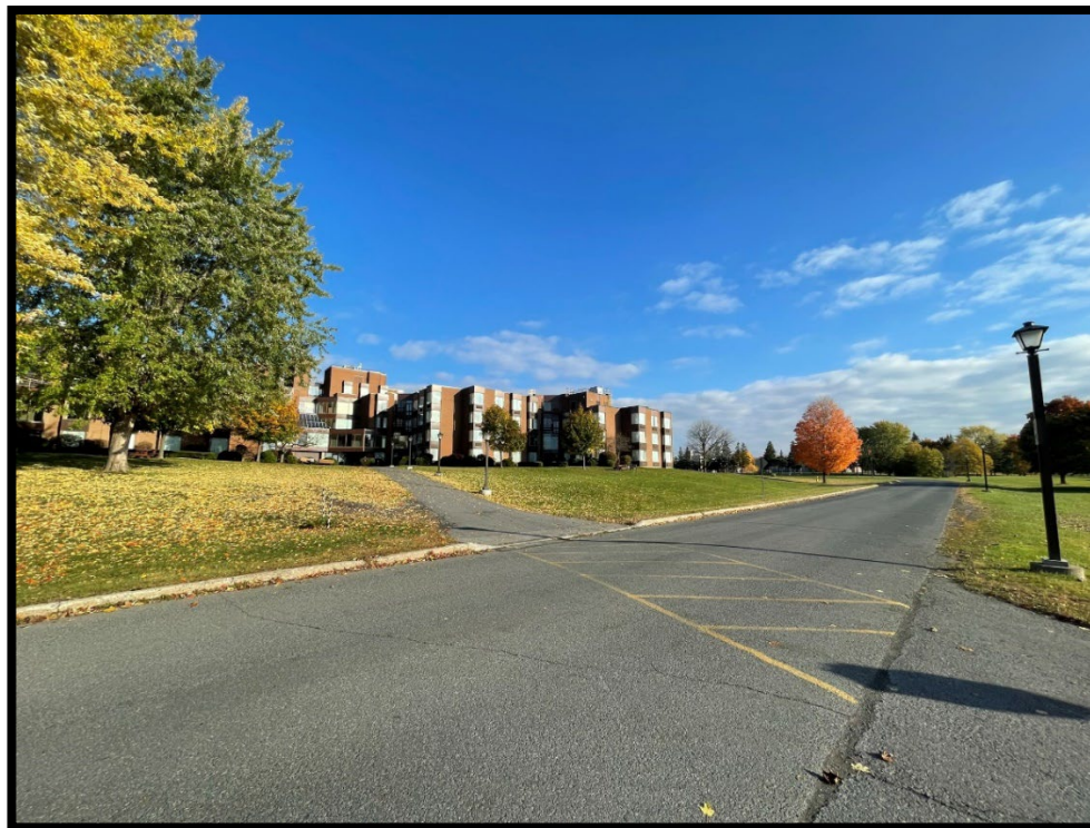
Figure 2: Roadway around hotel complex. (MH1136-D022)
