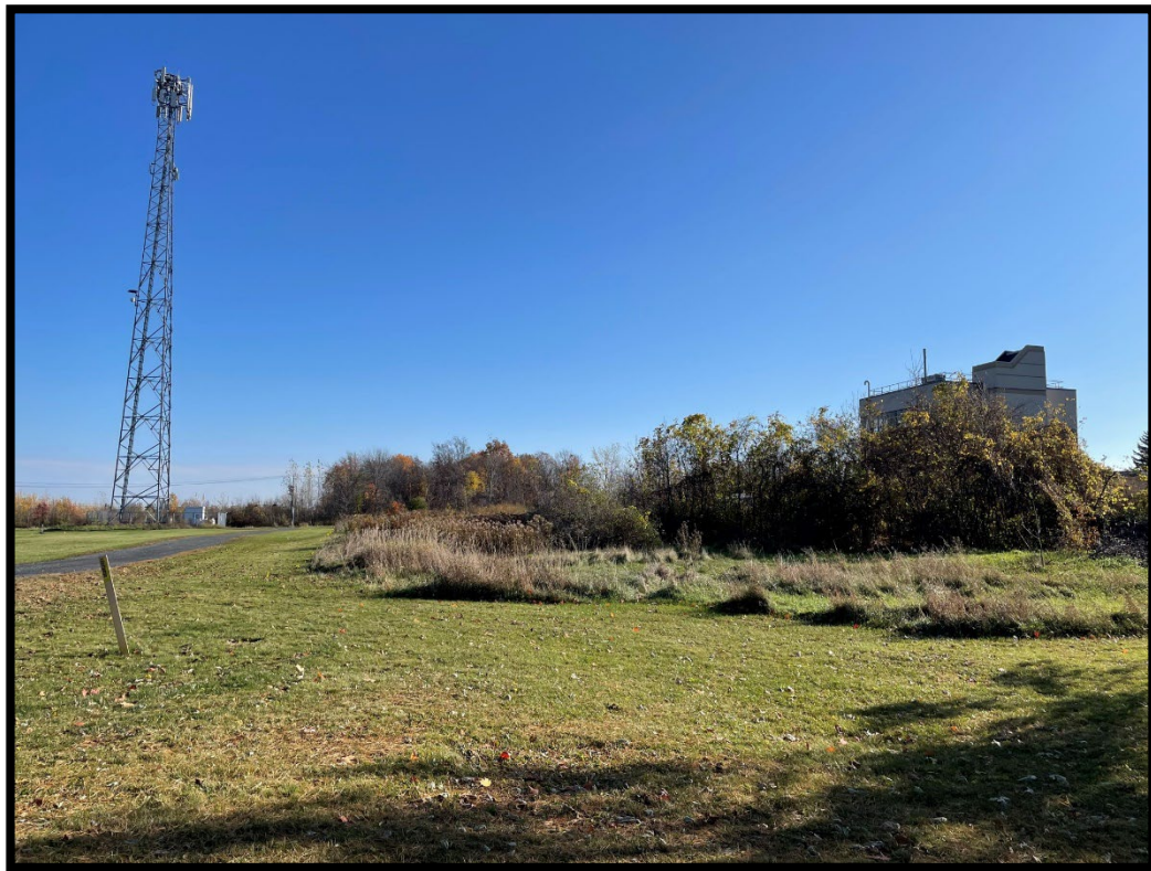
Figure 32: Edge of water treatment plant and cell tower. (MH1136-D045)
