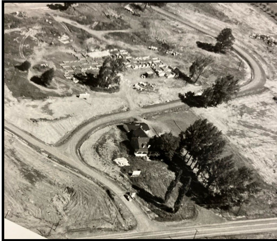
Figure 1: Historical limestone house just south (below) ongoing construction activity for the Transport Canada Training Institute circa mid 1970s. Showing extend of earth moving associated with the front lawns and gardens of the facility (provided by proponent).
