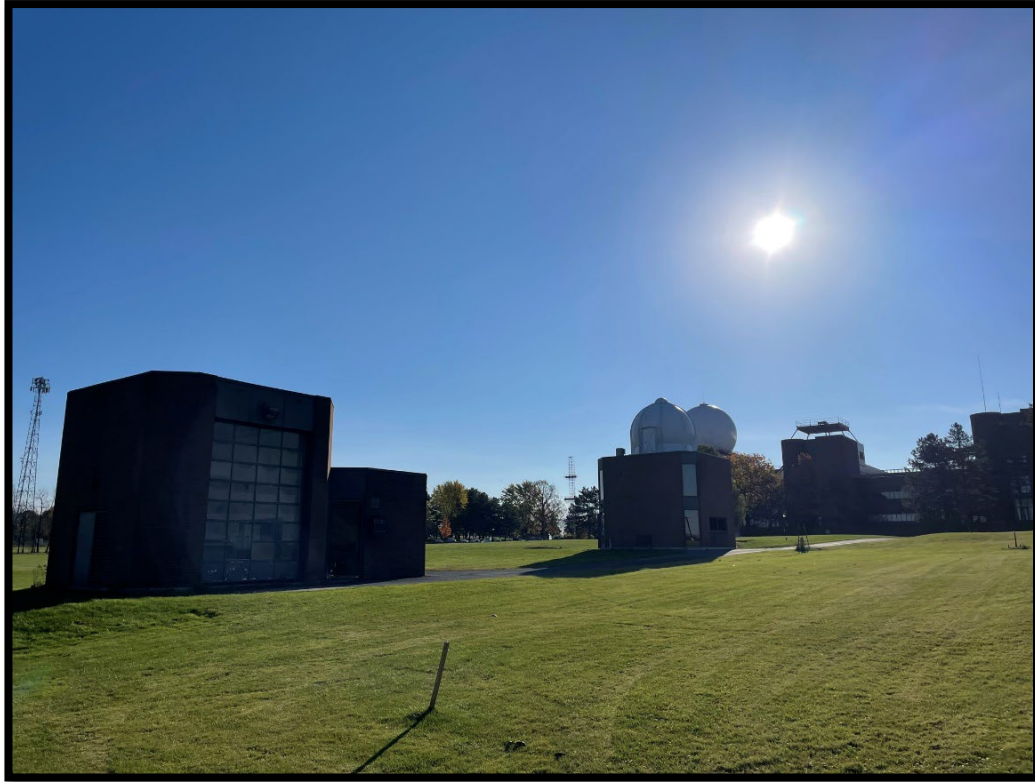
Figure 25: Monitoring and observation installations and buildings on the eastern side of the study area. (MH1136-D037)
