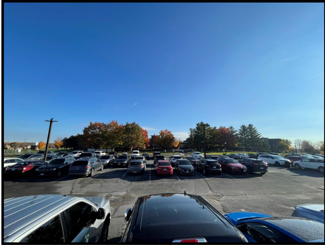
Figure 15: Parking lot in the northwest. (MH1136-D026)
