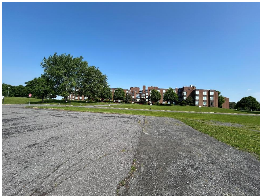
Photo 2 South side of Site Building A, June 10, 2025.
