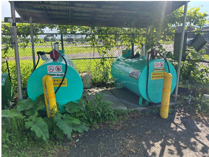
Photo 10 Two diesel ASTs in maintenance area northwest of Site Building A, June 10, 2025.
