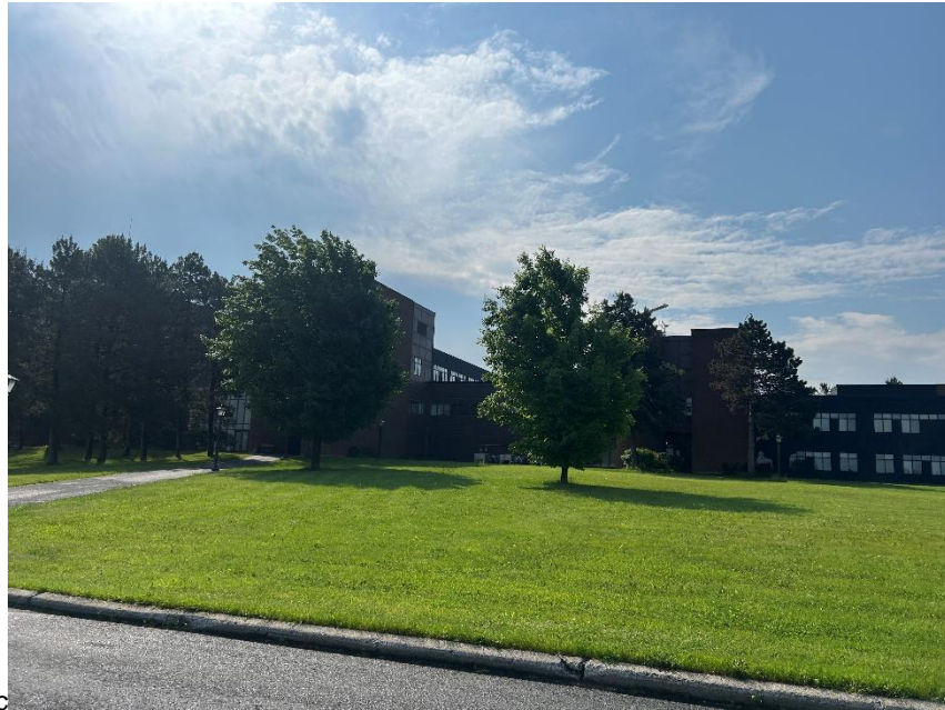
Photo 1 North side of Site Building A, June 10, 2025.
