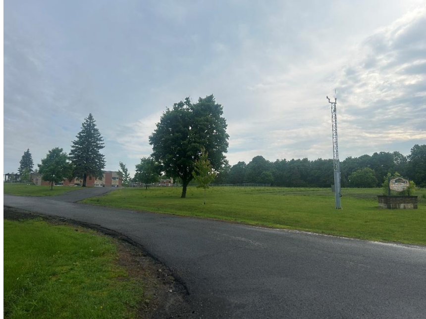
Photo 17 Properties east of the Site (waste water treatment plant), June 10, 2025.
