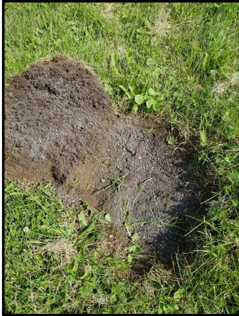
Figure 37: Disturbed soils under sod cap in northeast section – in progress (MH1184-D107).
