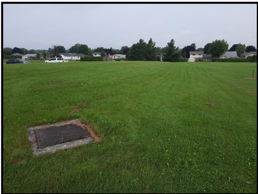
Figure 2: General conditions of northcentral lawn (MH1184-D018).
