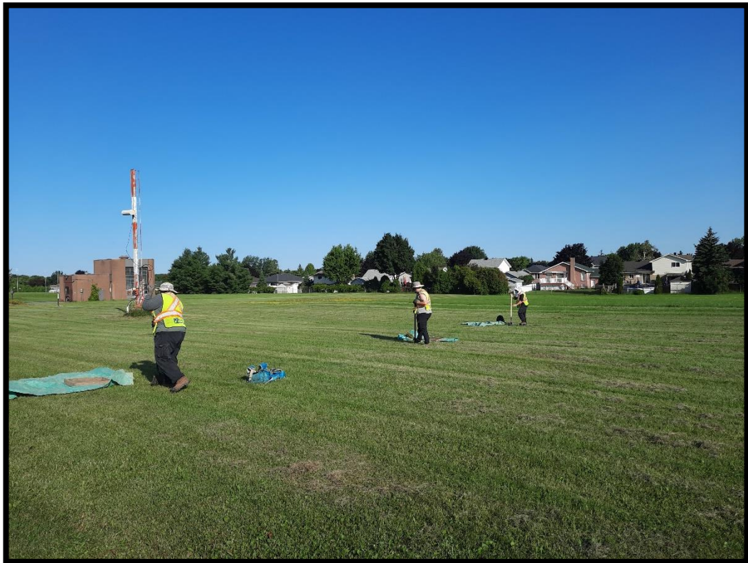
Figure 16: Test pitting in progress (MH1184-D026).
